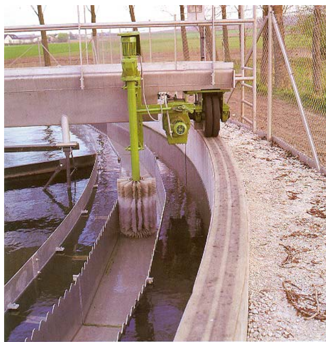
OUTLET CHANNEL CLEANING BRUSH DEVICE
